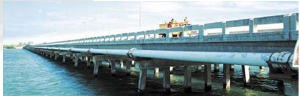
Longbird Bridge, Bermuda 58 years of protection by HDG rebar
