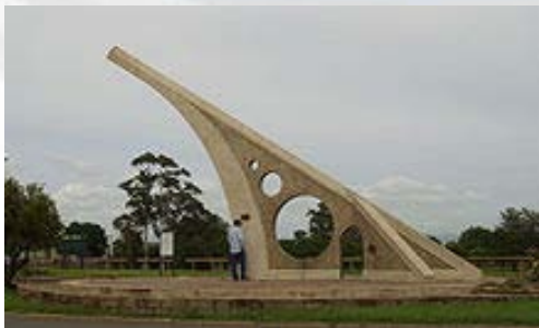
World's largest sundial Singleton NSW Australia 30 m 3 concrete, 2.5 T HDG rebar
